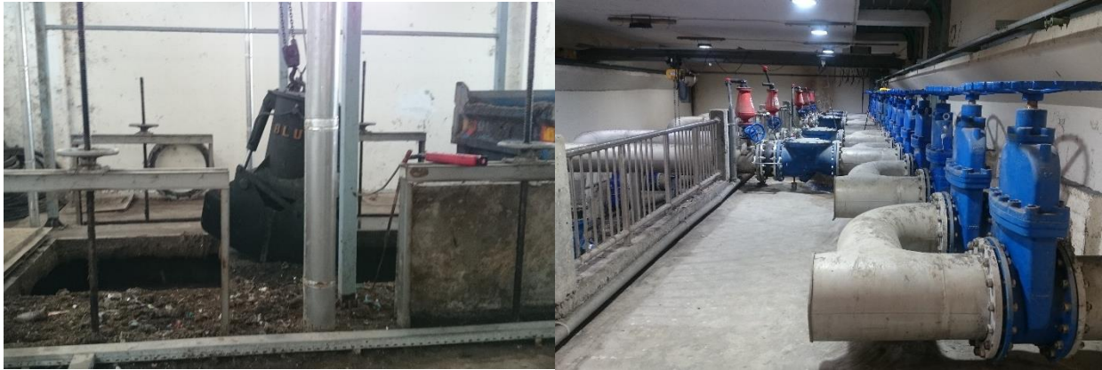
Figure 2-5: Sites for rehabilitation works at the TPS location
