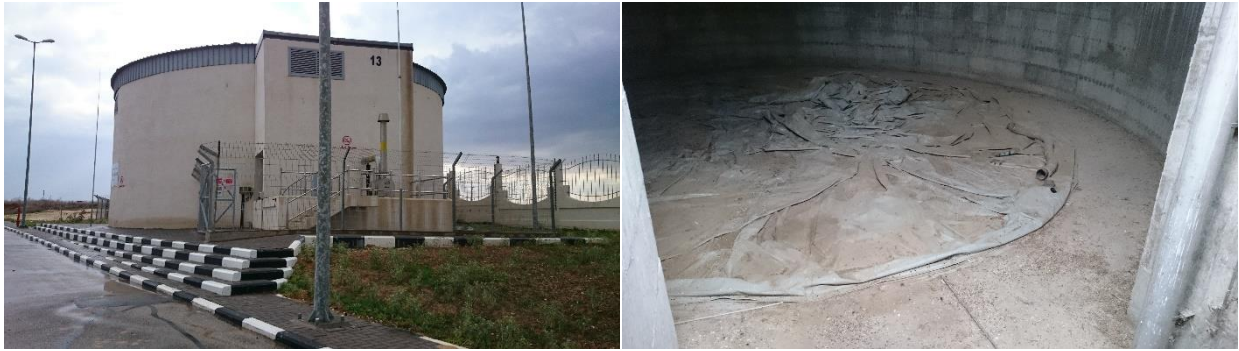
Figure 2-2: The biogas balloon site at NG WWTP
